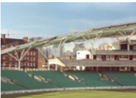
FAST BUILD TERRACING
