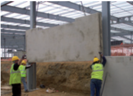
FAST BUILD GROUND BEAMS
