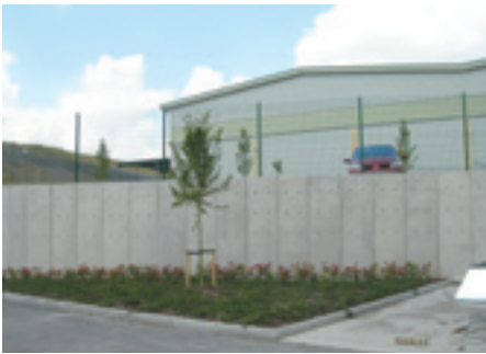
FAST BUILD WALLS
