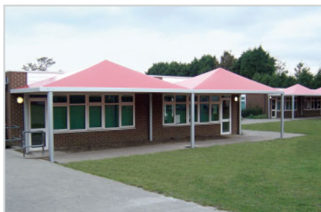
Apex roofs are very popular for buildings with flat roof lines.
