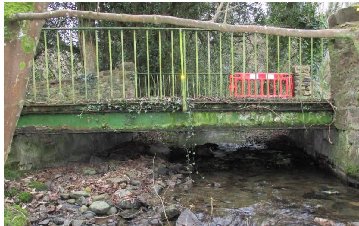
Bespoke deck and substructure replacement
