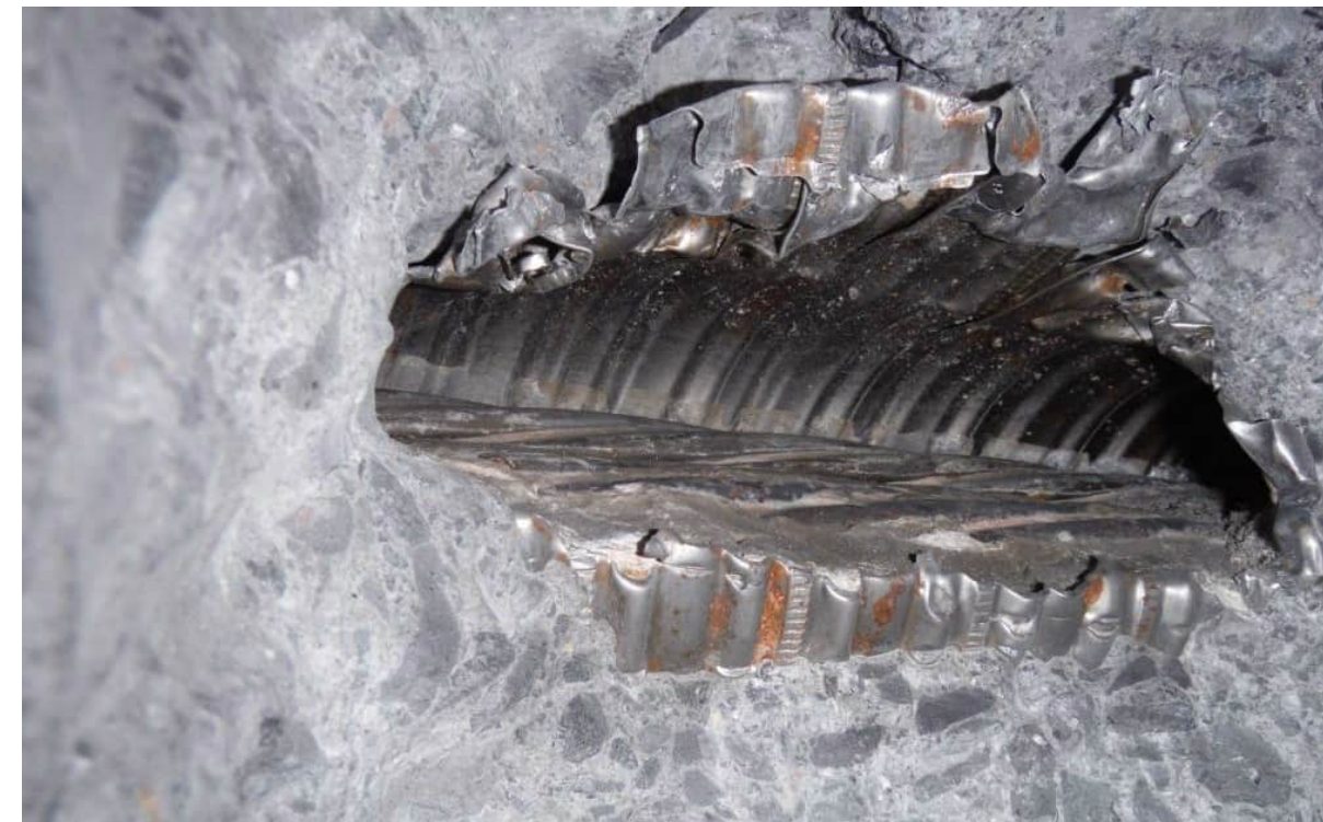
PTSI Inspections & Investigations
