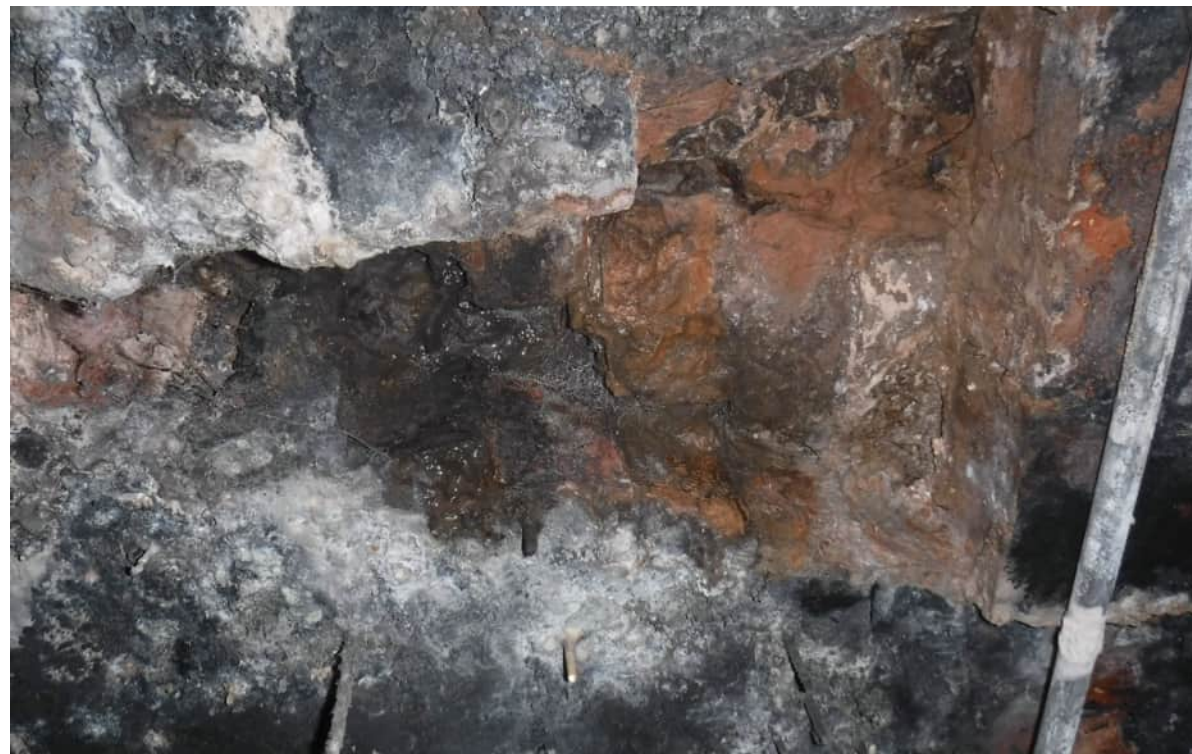
Masonry arch repairs
