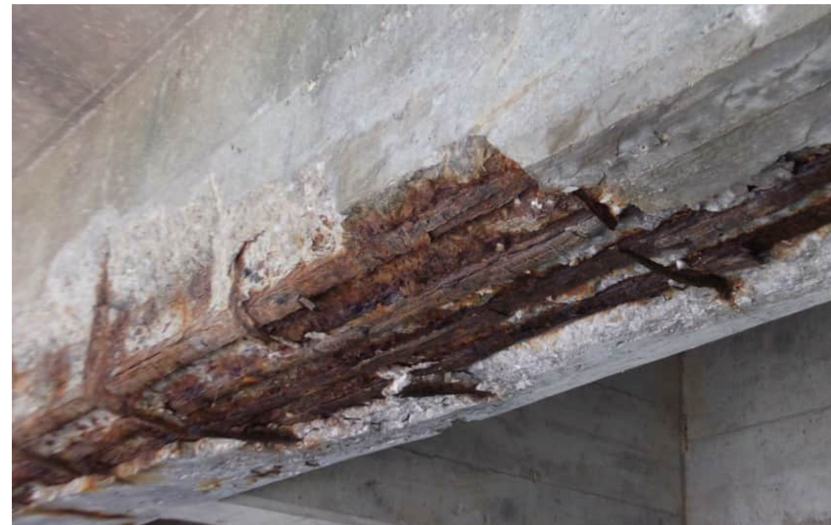
Reinforced concrete repairs
