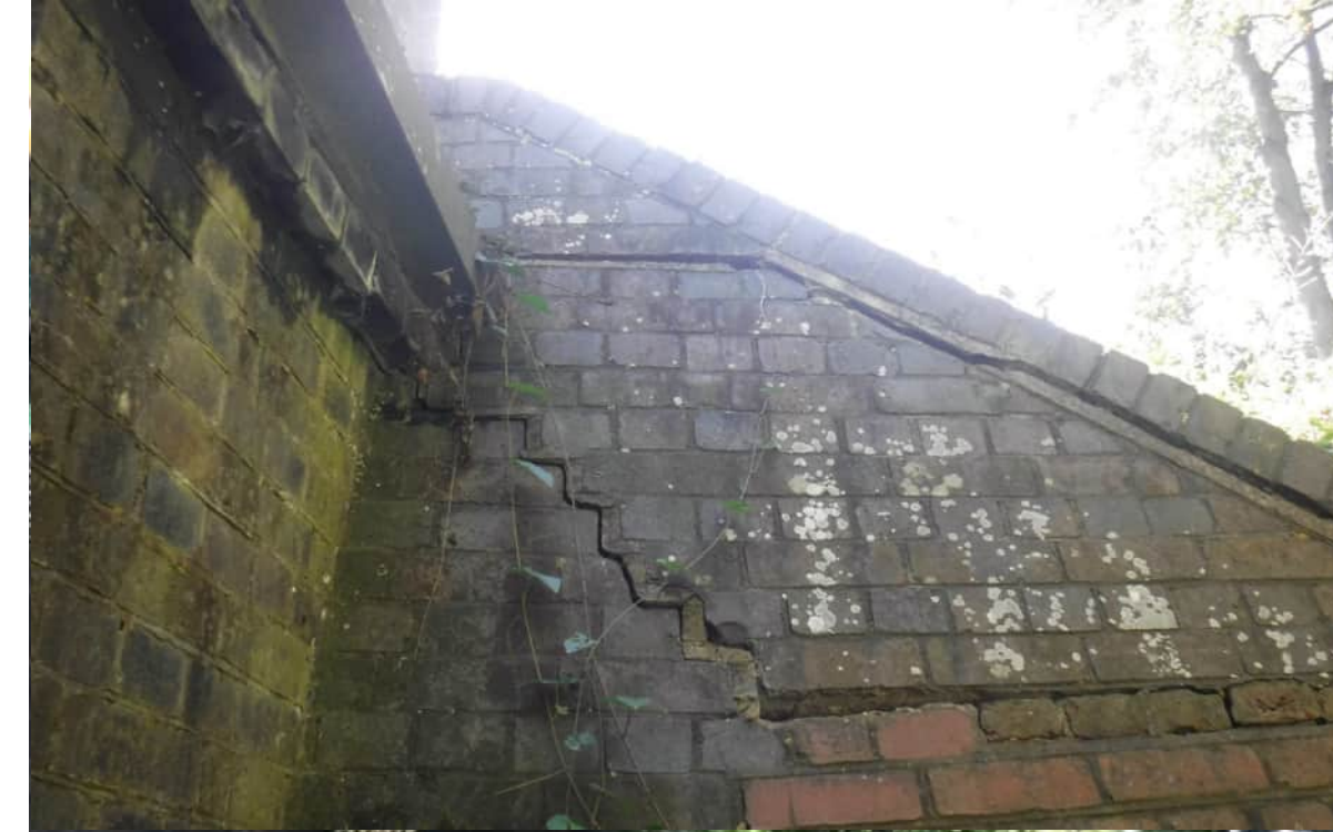
Substructure movement
