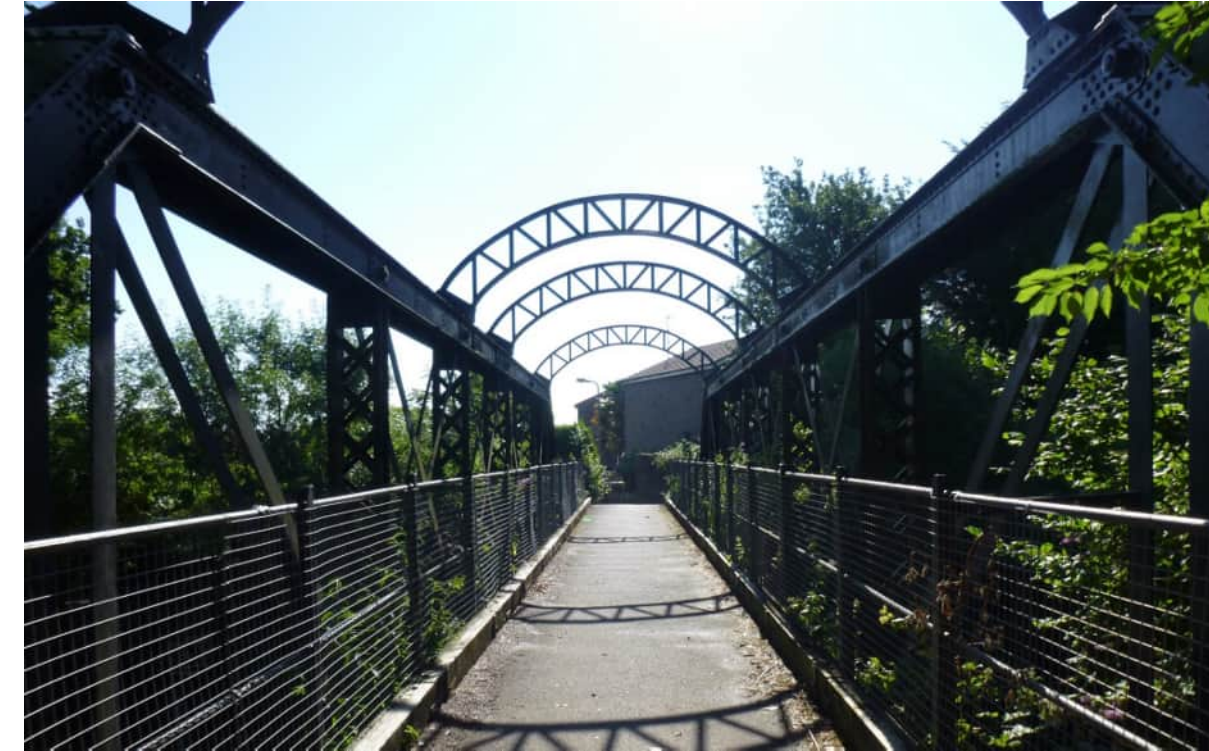
General & Principal Inspections (DMRB)
